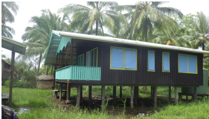
A new, but unopened health clinic built in Gulf Province with funding from the District Service Improvement Program.
