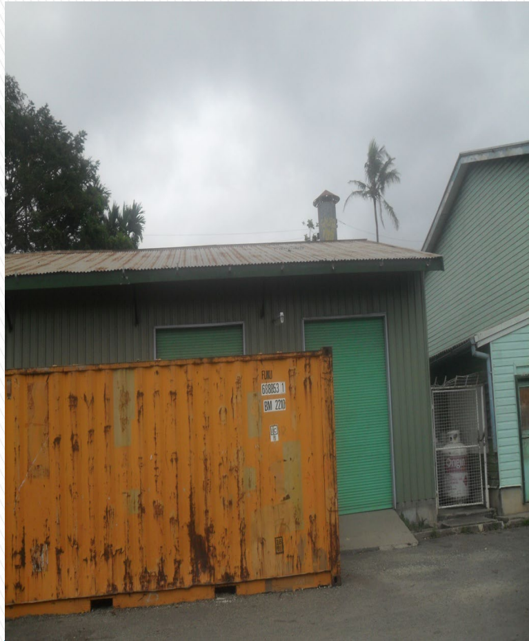
Medical waste incinerator in POM General Hospital
