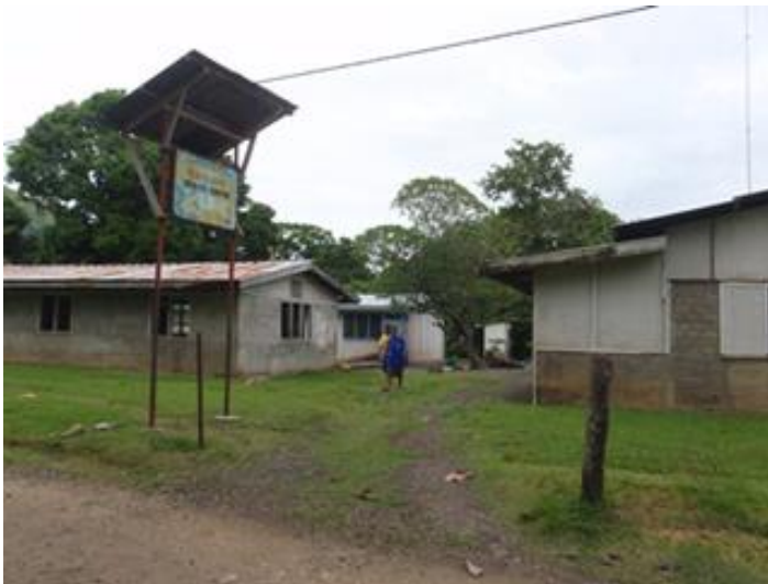
Photo: rural health facility, Milne Bay Province (source: Watson)
