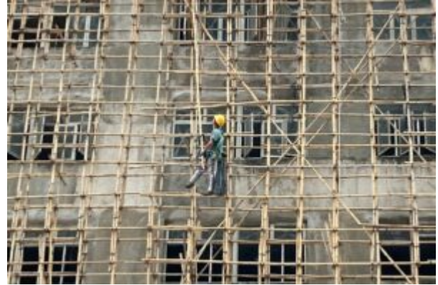
Bamboo scaffolding at a construction site Photo Credit: Unsplash/Thomas Kinto
