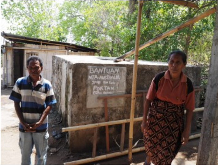
A concrete water tank constructed in Flores.
