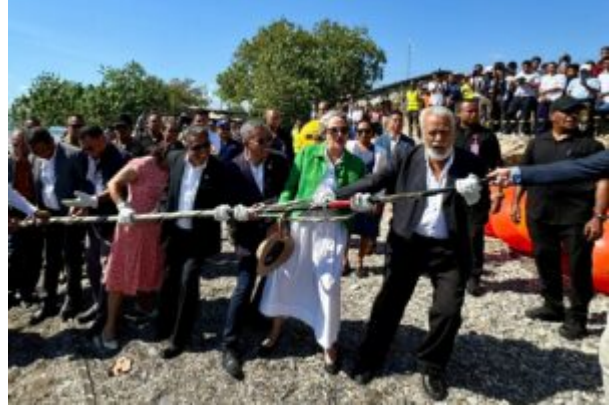
The launch of the Timor-Leste South Submarine Cable at Bebonuk, June 2024
