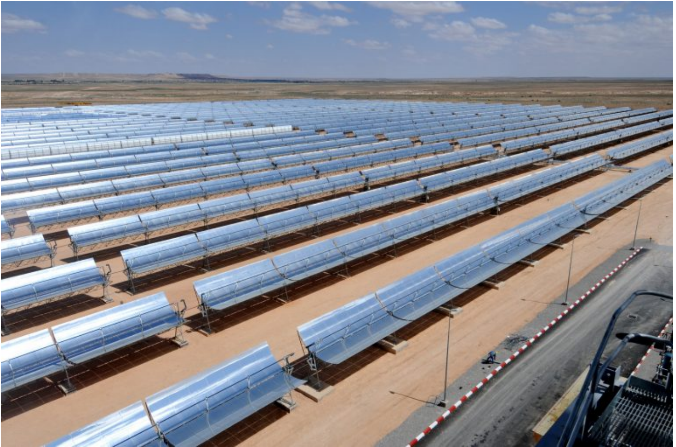
Thermo-solar power plant ( Dana Smillie/World Bank/Flickr )
