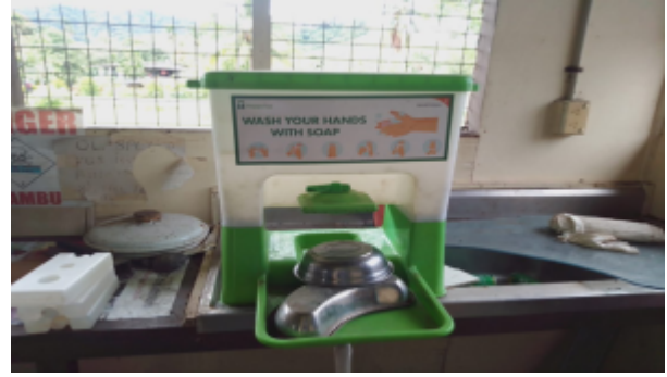
Bogia District Hospital, Madang Province, Papua New Guinea
