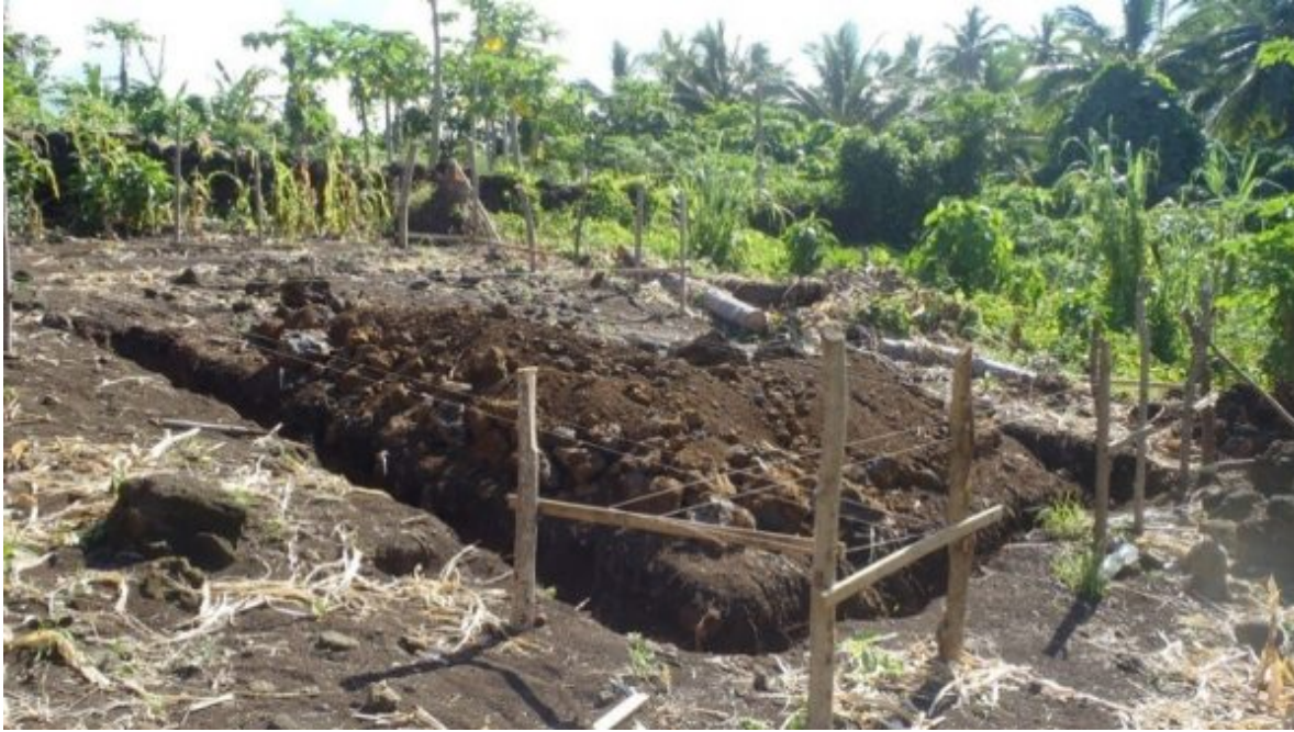
Chez Maureen Bungalows (before building)
