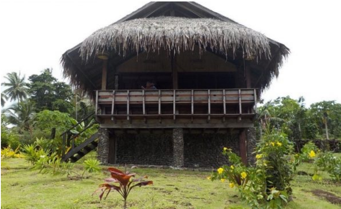
Chez Maureen Bungalows (after completion)
