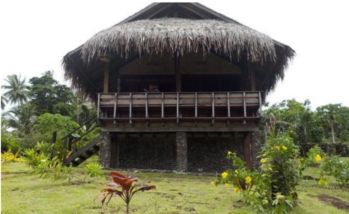
Chez Maureen Bungalows (after completion)
