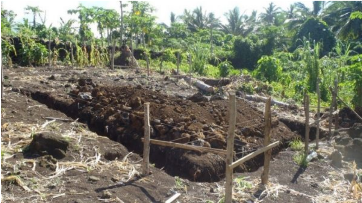
Chez Maureen Bungalows (before building)
