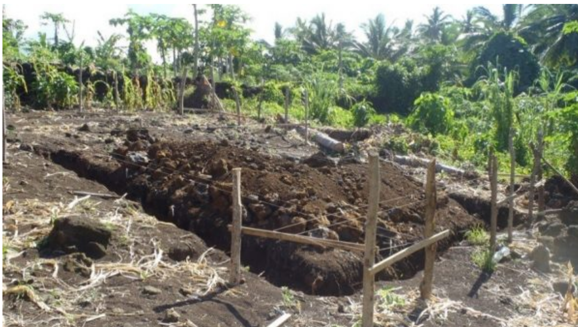
Chez Maureen Bungalows (before building)
