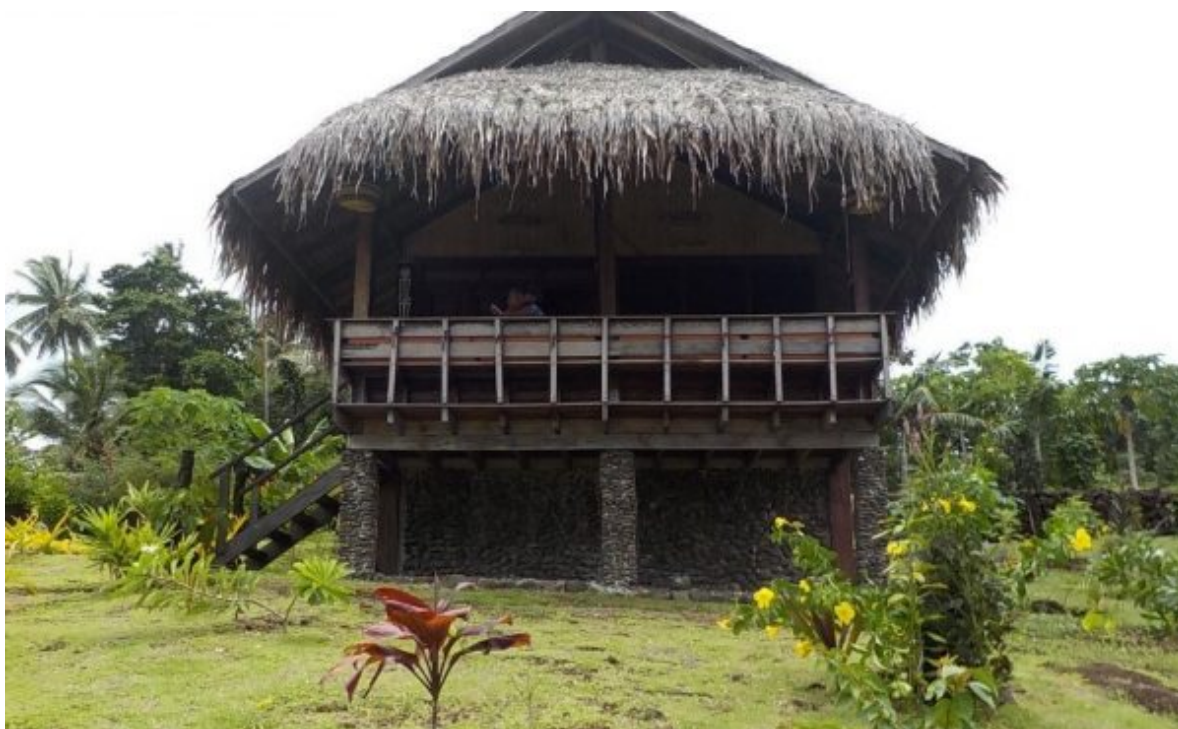
Chez Maureen Bungalows (after completion)
