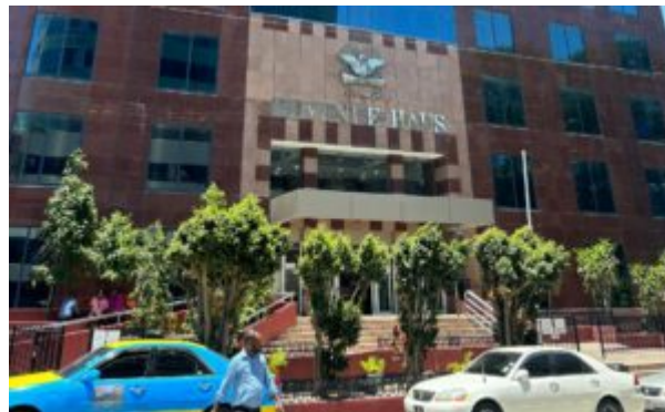
Revenue Haus in Port Moresby is the headquarters of Papua New Guinea's Internal Revenue Commission.
