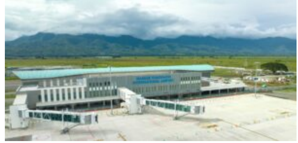
Nadzab Tomodachi International Airport in Morobe Province, Papua New Guinea
