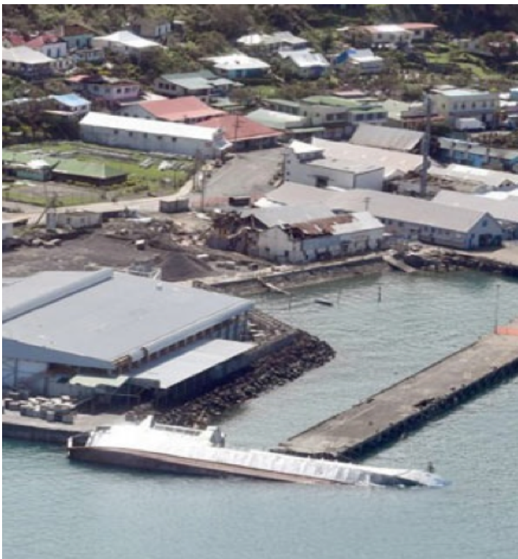
Cyclone Winston damage at Levuka (Photo: New Zealand)
