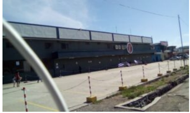
TST Waigani shop during shut down (taken by author)
