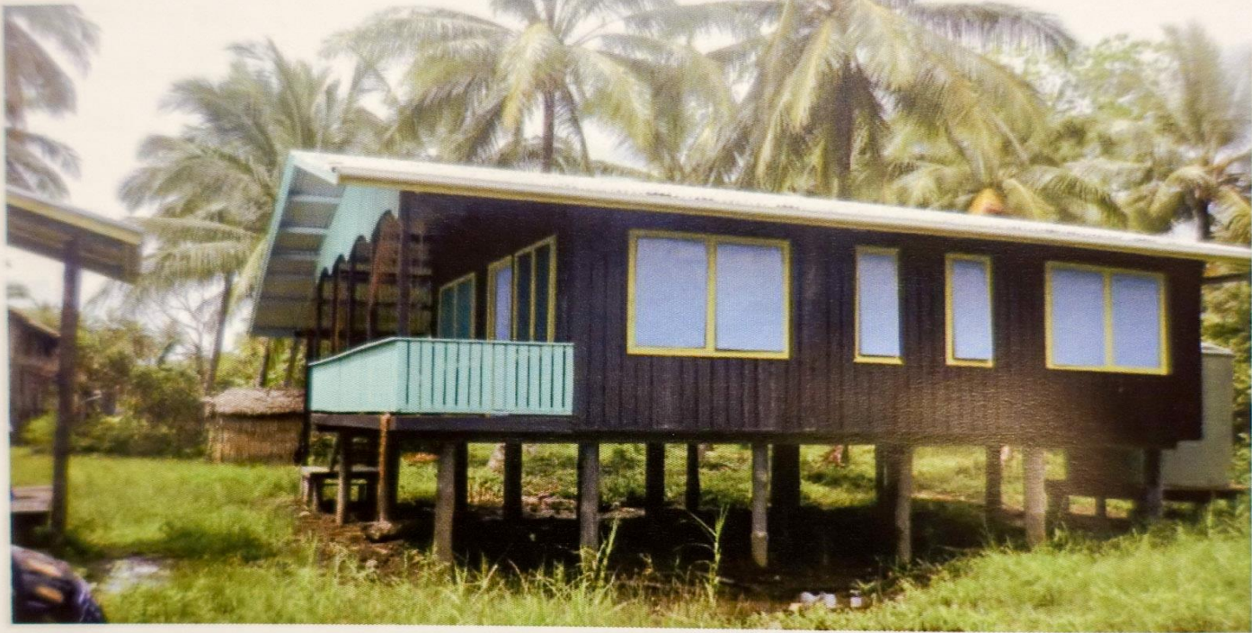
A new, but unopened health clinic built in Gulf Province with funding from the District Service Improvement Program.
