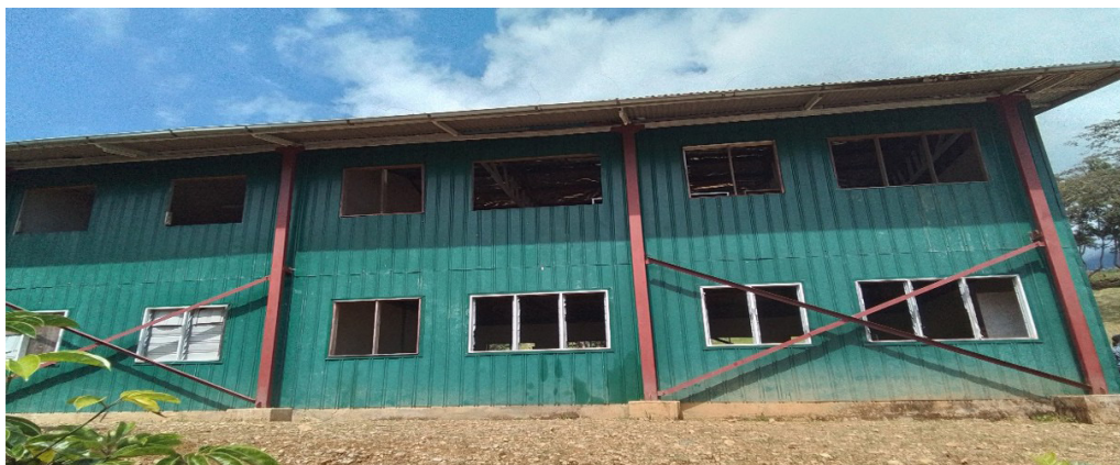
Incomplete new classrooms, view from the back, June 2024 (Rex Kupil)
