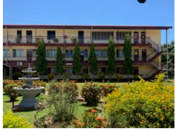
A school stands empty in Fiji Photo Credit: Neelesh Gounder
