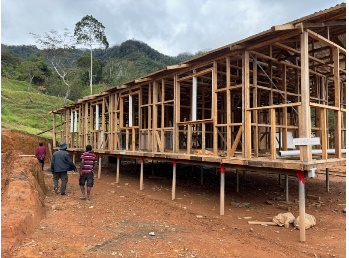
Health centre under construction at Hawabango.
