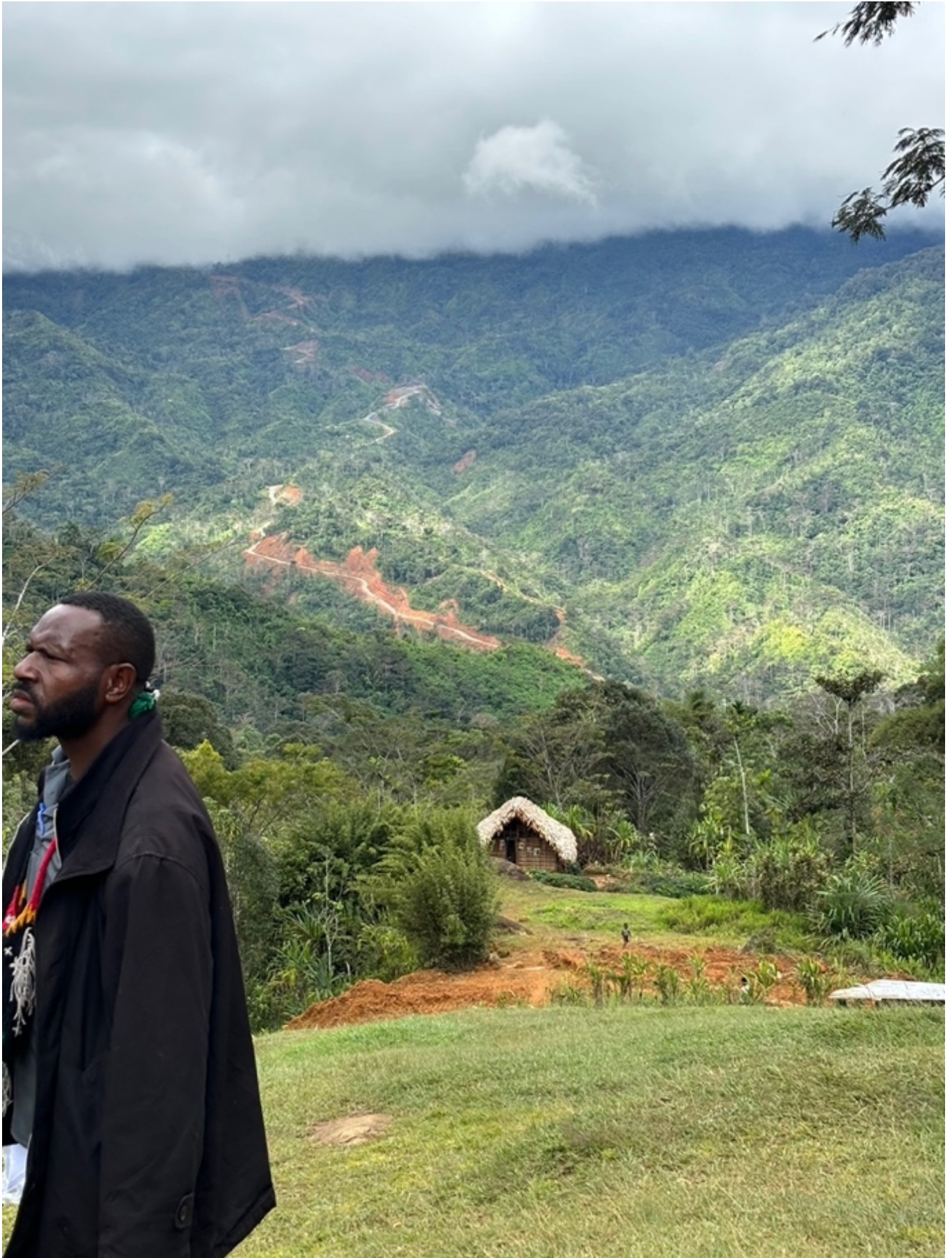
The Connect PNG road cut into the mountainside above Bema station.
