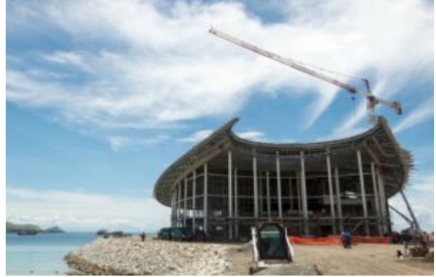
APEC Haus during construction. ONEPNG News
