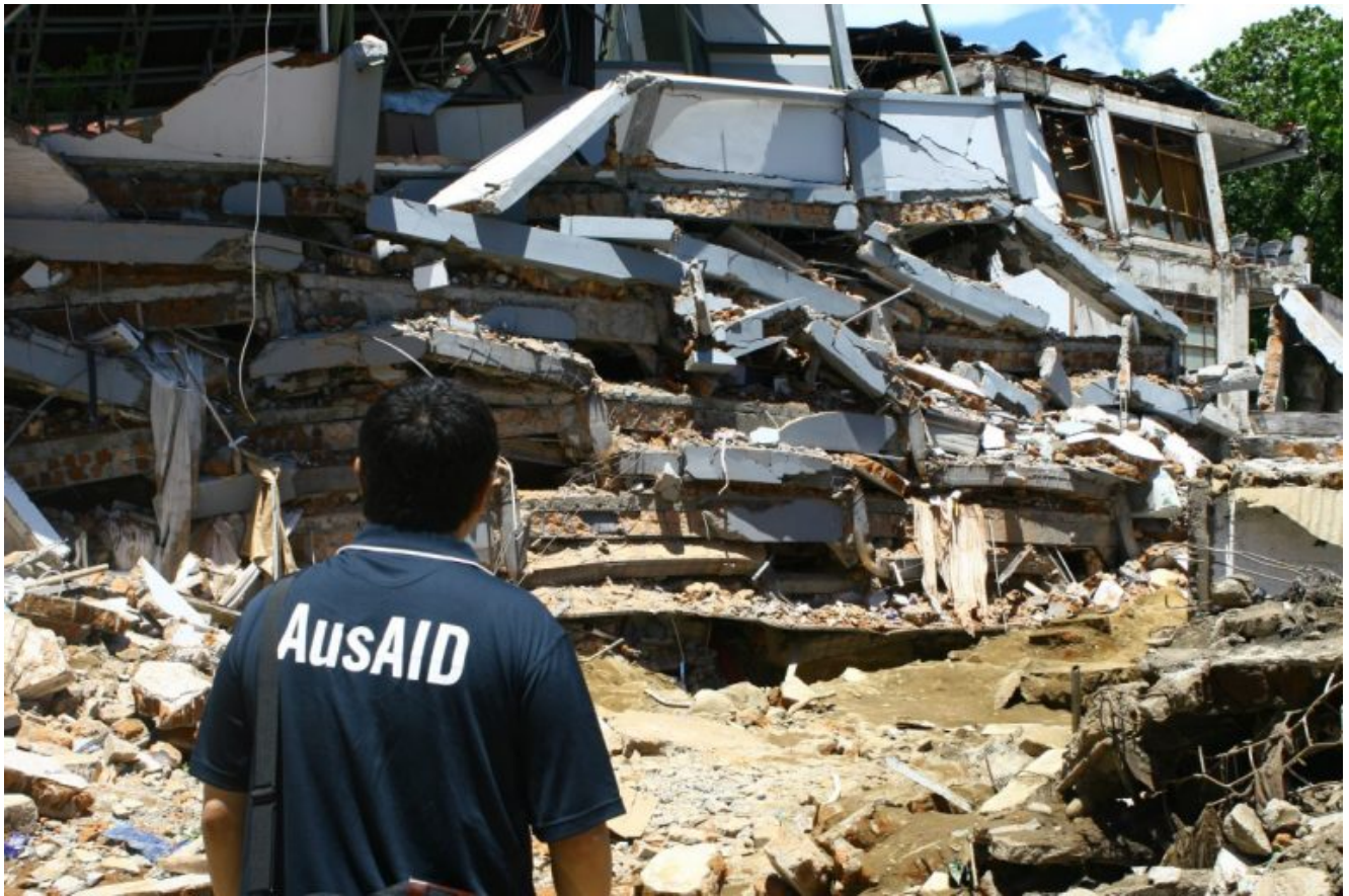
AusAID response to the 2009 Padang earthquake, Indonesia. ( DEAT/Flickr )
