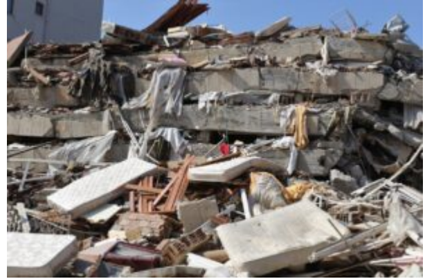
Earthquake destruction in Antakya/Hatay in Türkiye
